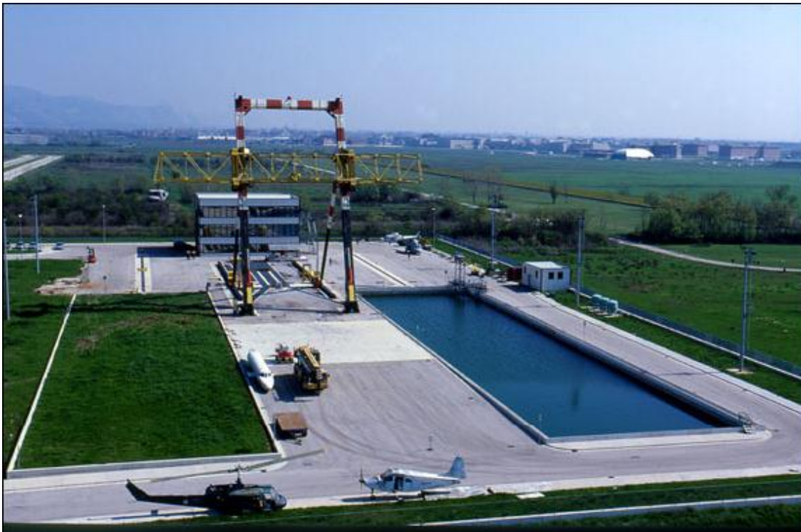
Figure 1: General view of the facility with the 3 impact surfaces (soft, solid and water)
